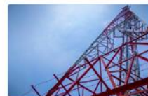
Telecom base station
